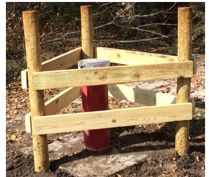
LLNRD monitoring well installed for Columbus Recharge Project
