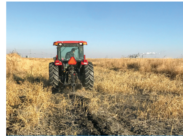
Discing the Lost Creek channel allows for groundwater infiltration.
